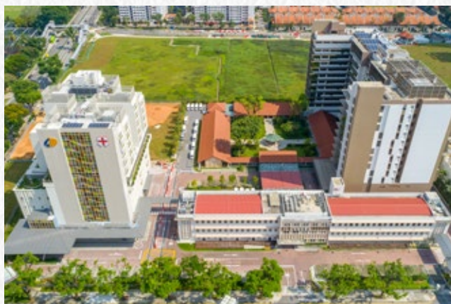
Block F on the left houses the new wards while the existing nursing home building Block B is on the right. 新病房坐落在F座大楼（左）内而图中右侧则是本院现有的疗养院大楼（B座）
